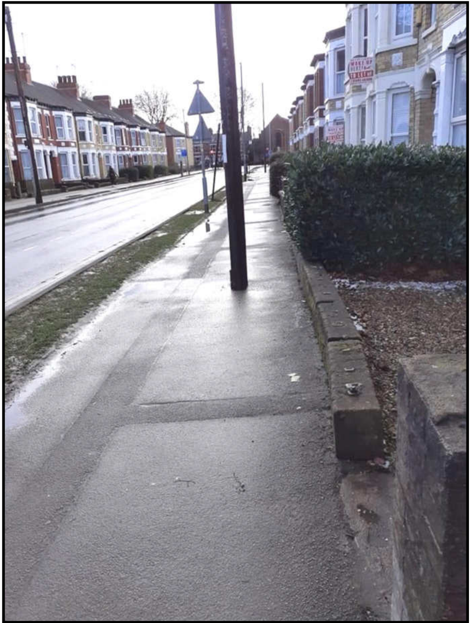
A POLE PLANTED IN THE CENTRE OF THE FOOTPATH, DANGEROUS AND AN OBSTRUCTION
