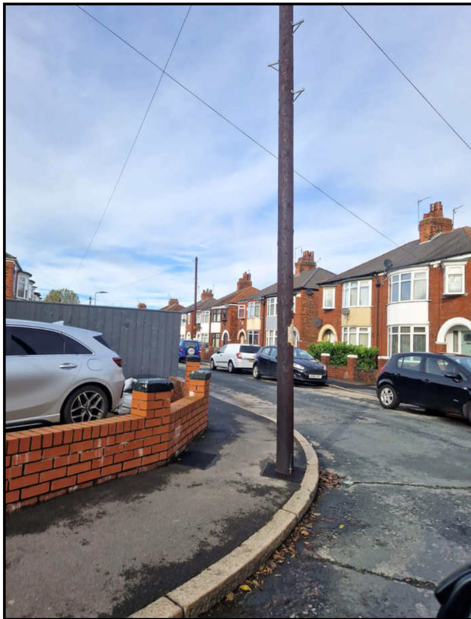
A POLE PLANTED ON A CORNER AT THE EDGE OF THE ROAD OBSTRUCTING DRIVERS VIEW
