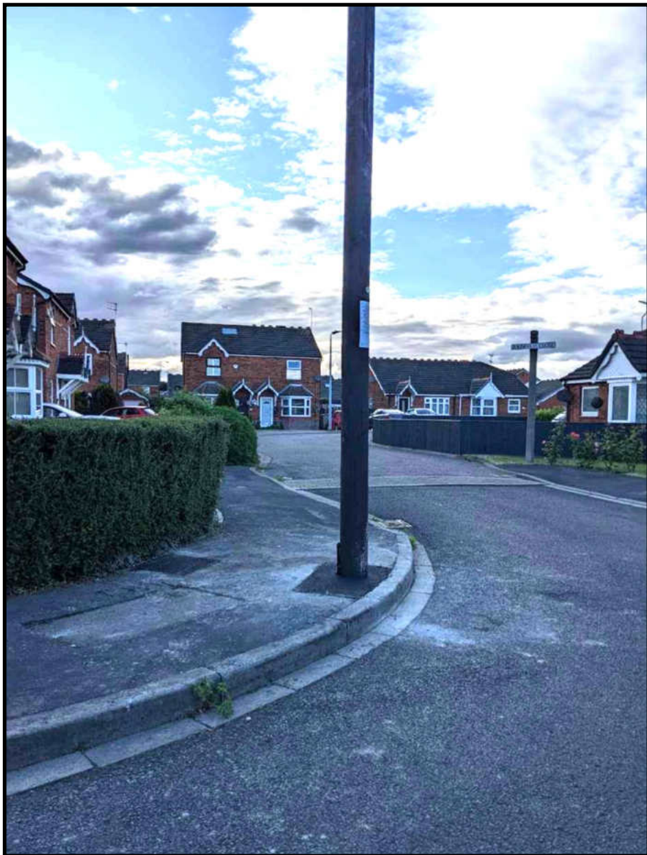
A POLE PLANTED ON A CORNER AT THE EDGE OF THE ROAD OBSTRUCTING DRIVERS VIEW
